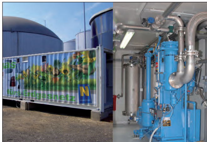
Figure 3: View of the shipping container used for the membrane up-grading equipment (left) and the membranes themselves inside the container (left side of right photo).
