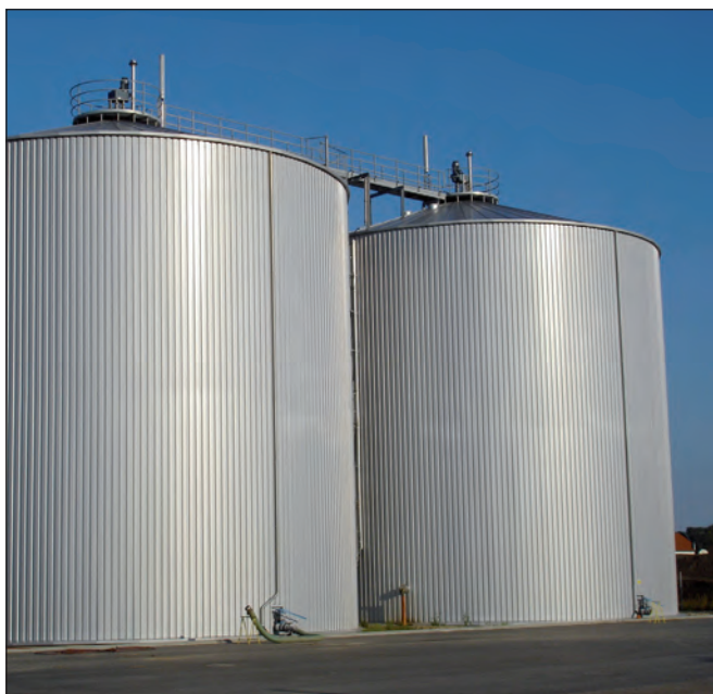
Fig. 1b: General photos of the Bruck an der Leitha biogas plant
